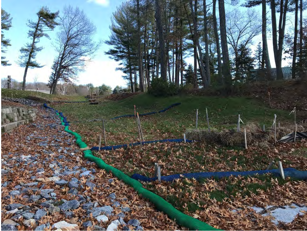
Fig 3: Slope above the manhole at Gundalow Landing/east side of the bay. Viewing east. (11-24-20)
