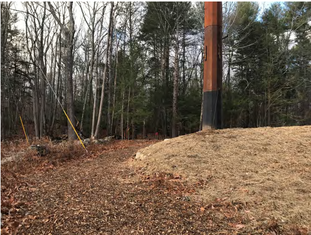
Fig 8: Str. 90 work area. Viewing southwest. (11-24-20)
