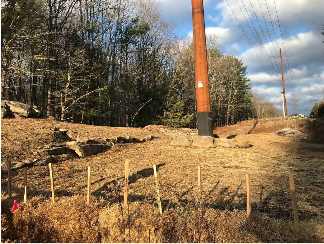
Fig 7: Str. 89 work area. Viewing northwest. (11-24-20)
