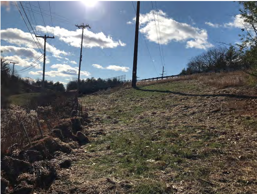
Fig 12: Str. 6 work area. Viewing southeast. (11-24-20)
